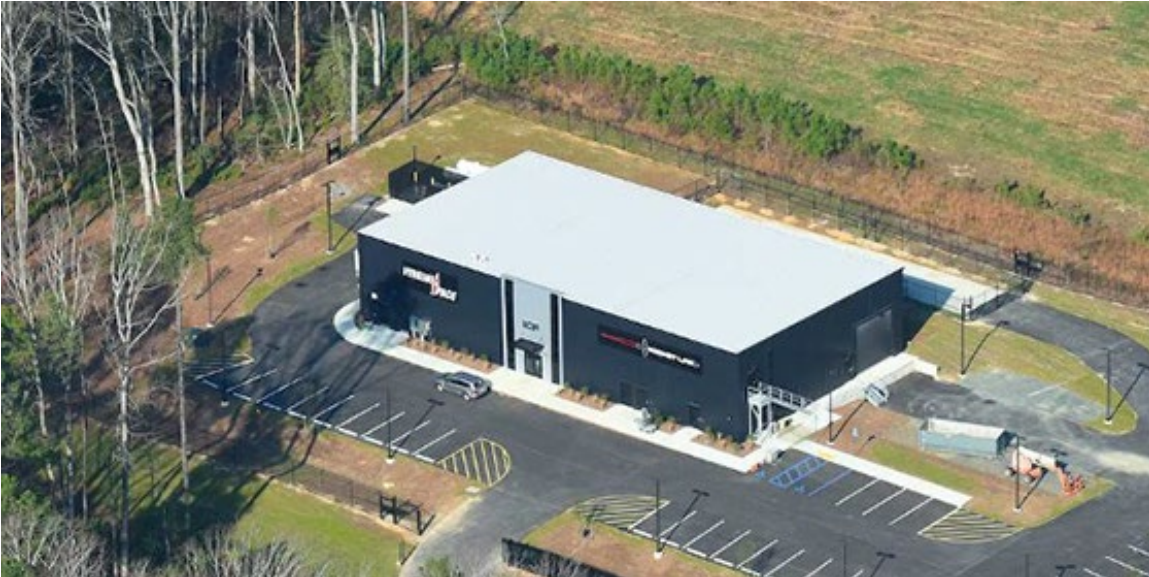
Figure 90: Integration and Control Facility (ICF)
