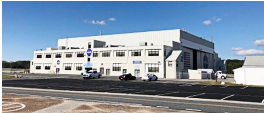
Figure 74: Aircraft Operations Hangar (Building D-1)
