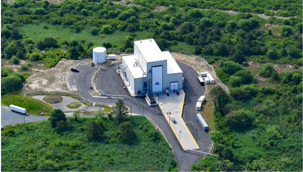
Figure 85: MARS Payload Processing Facility
