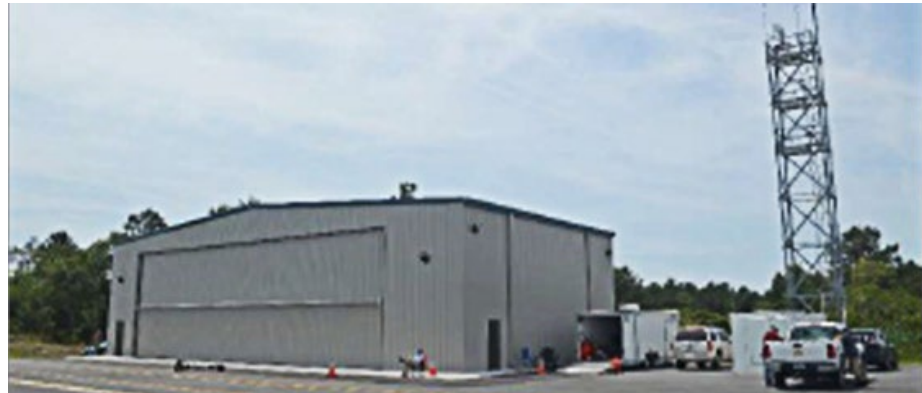
Figure 83: MARS UAS Airfield Ramp Area
